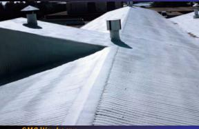
SPF is equally well suited for metal roofs. SPF can be applied directly to the metal surface, whether bare galvanized or pre-coated panels.
