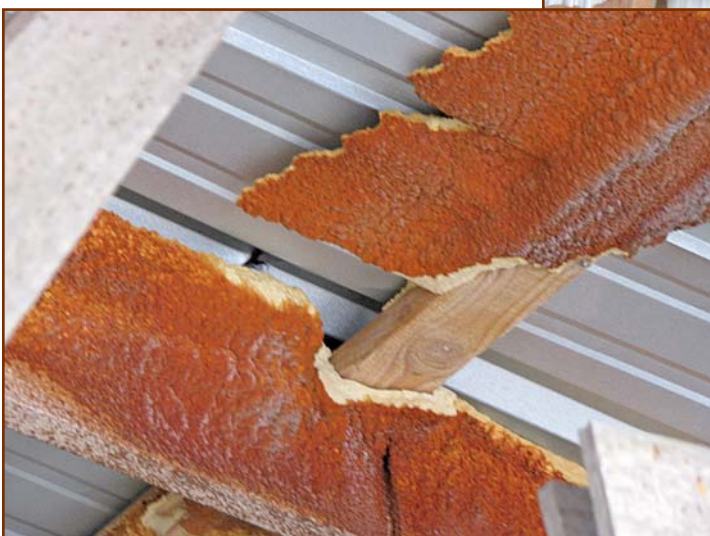
Figure 6 – The ccSPF was removed to install new metal.
