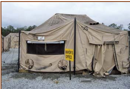
Photo 16 – Example before application of ccSPF.
