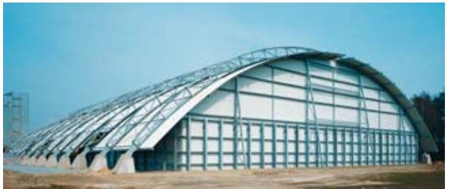
△▷ This 16,000 m 2 grain store in Essen, Oldenburg, with an external steel skeleton construction is thermally insulated from the inside and made airtight: with Elastopor H.
