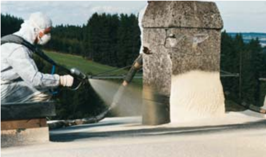
◁△ Jointless insulation and sealing with Elastopor H for buildings old and new.
